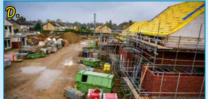
Project: De Srijeners
